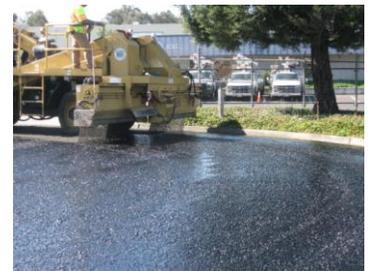
**Chip seal operation in progress**
