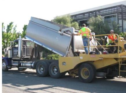
*Loading rock "chips" in the spreader*
