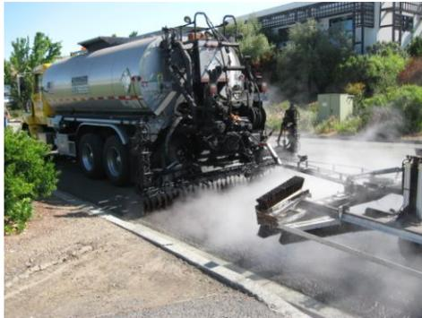
*Placing oil on prepared road surface*
